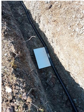
Cables are positioned inside a small trench
