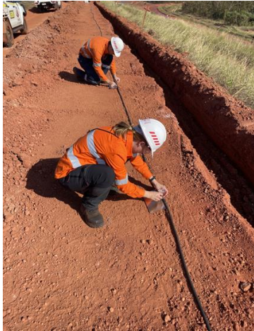
Cables are positioned inside a small trench
